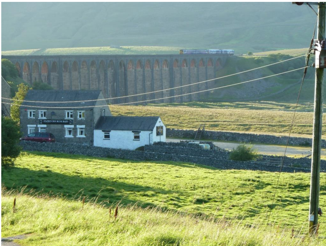
The homeward bound DalesRail train crossing Ribblehead Viaduct on 22 nd August 2010 - Richard Watts
