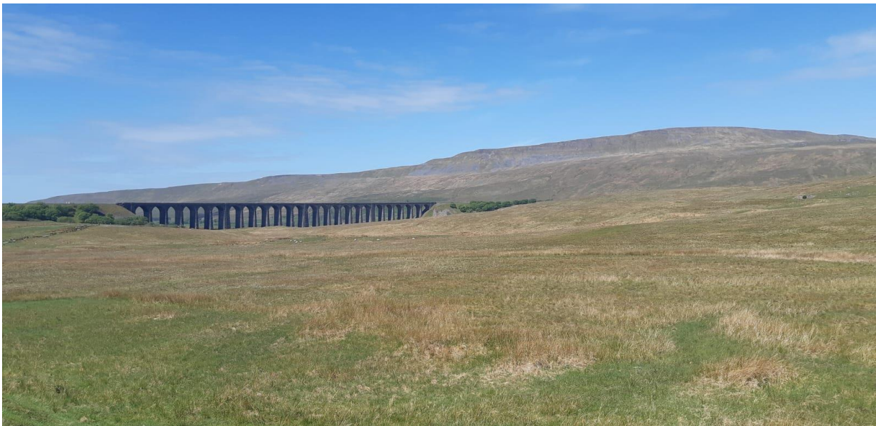
Ribblehead Viaduct looking towards Whernside – Chris Watts
