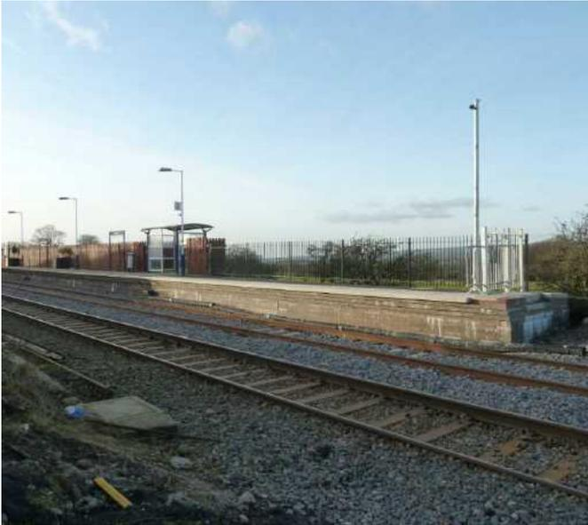
Since the last issue of Reading Between The Lines, Network Rail have completed the work to extend the platforms on the stations on the Clitheroe Line. The project was part of the Government's HLOS (High Level Output Specification) and will allow the stations to cope with the strengthened service now running in the morning and evening peak periods.
