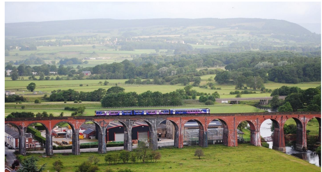
Whalley Viaduct with Stonhurst College in background
